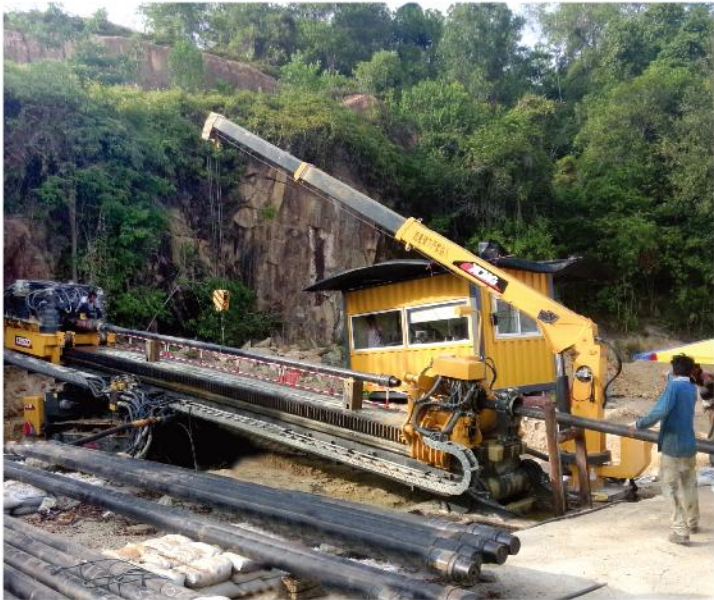
XZ5000在马来西亚穿越卢穆特海湾 XZ5000 works to get through Lumut Bay in Malaysia
